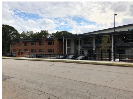
1). North Elevation - Jan 13, 2020
